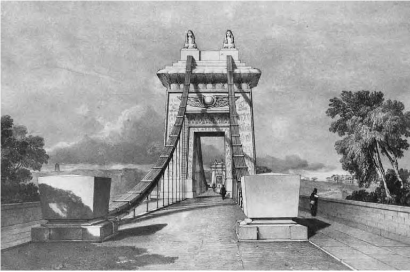
Plate 159 Gateway (actually the pylon-tower from which the structure is suspended) to Clifton Suspension Bridge, 1831. Lithograph after the unrealised design by Isambard Kingdom Brunel. The pylon was derived from that at Dendera, but the pylon-form is admirably suited to suspension-bridges, while, extended, the battered form is ideal for retaining-walls, dams, and the like, so similar shapes are found in many structures of the nineteenth century. Note the pylon-piers with winged globes, sphinxes on top, battered opening and sides, and the cables anchored in massive sarcophagi-like blocks (City of Bristol Museum and Art Gallery).
